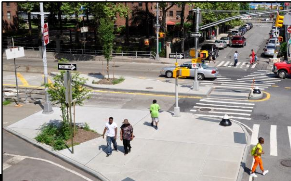
Concrete neckdown/extension example
