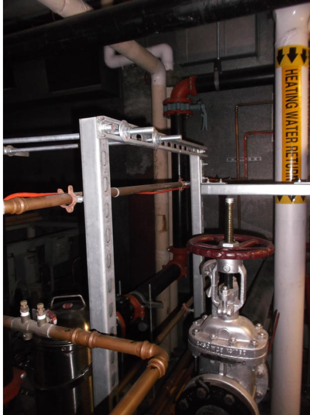
Hot water feed up to 2 nd floor mechanical room
