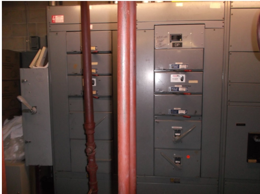
Electrical Equipment Located Adjacent to Boilers
