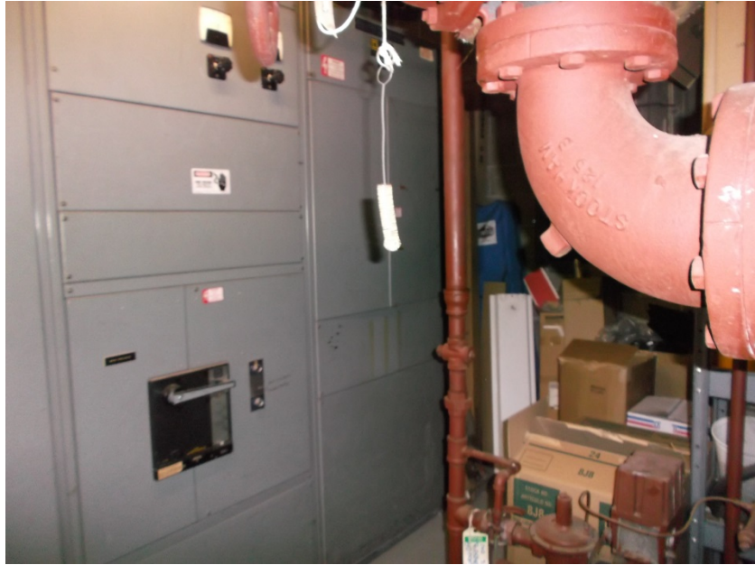
Electrical Equipment Located Adjacent to Boilers
