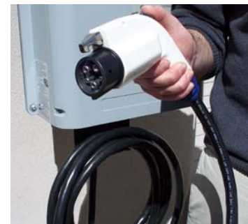
Figure 6-6. EVSE Level 2 charging equipment with a SAE 1772J connector. Photo by Angela Costanzo, NREL/PIX 18723
