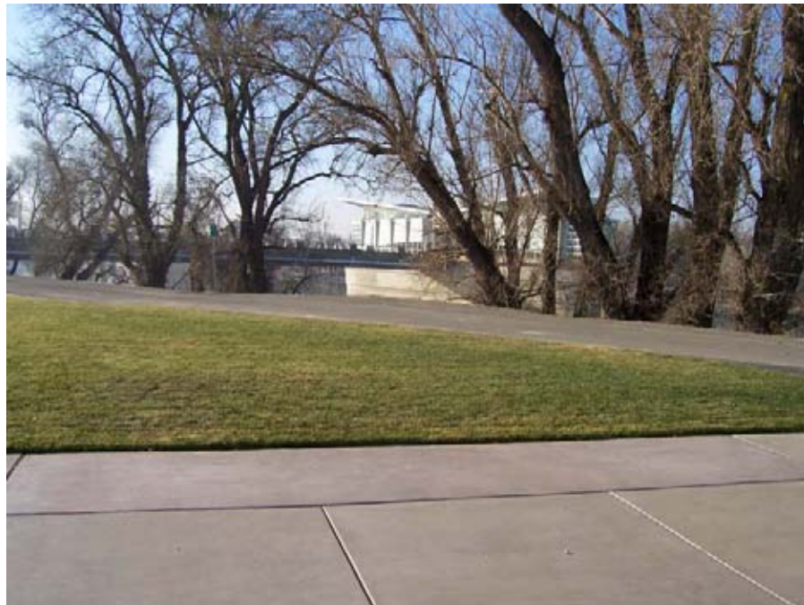
Water Supply intake structure in Sacramento River directly west of Jibboom Park.
