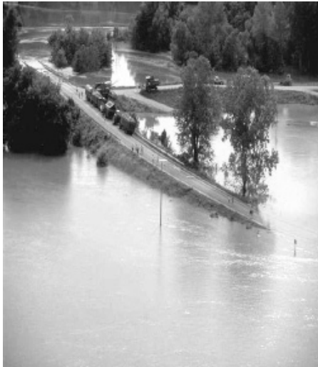
Following a disaster, repairing major roads is a high priority among short-term recovery tasks.
