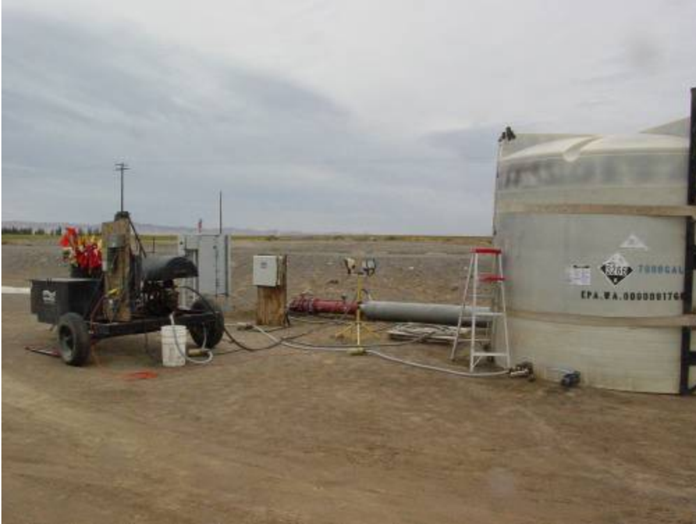
Chemigation injector trailer and bulk nurse tank
