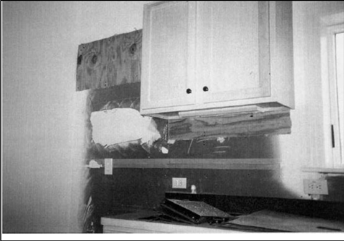
Photo 11: Dominion Building Group Site - Kitchen Cabinet Placement
