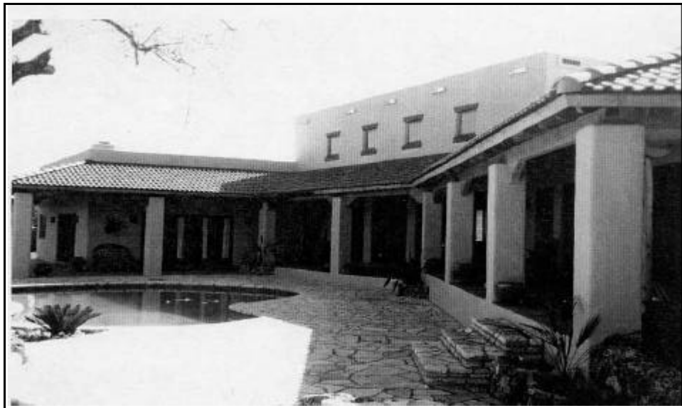
Photo 13: Site #2 - Rear Elevation
