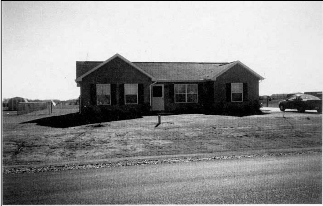
Photo 45: Site #4 - Front Elevation
