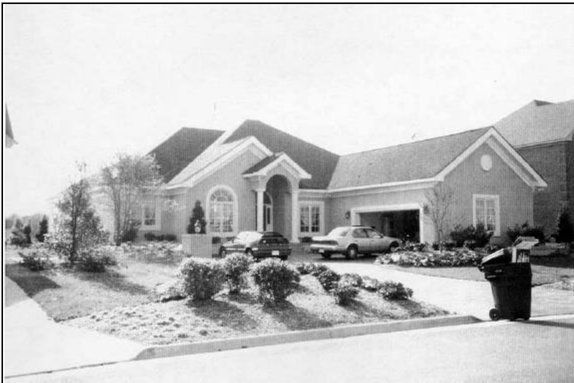
Photo 1: Site #1 - Front Elevation
