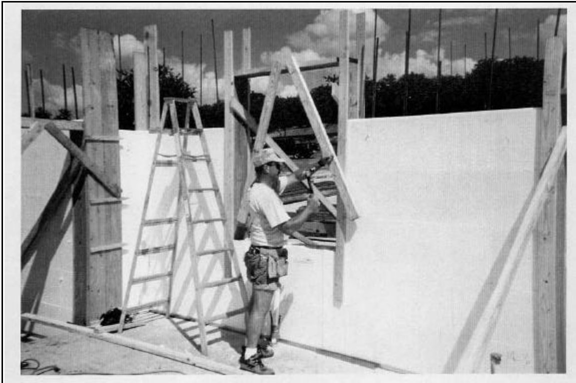
Photo 15: Site #2 - Window Jamb Construction
