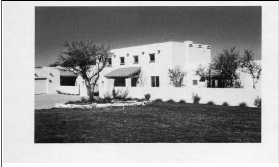
Photo 12: Site #2 - Front Elevation
