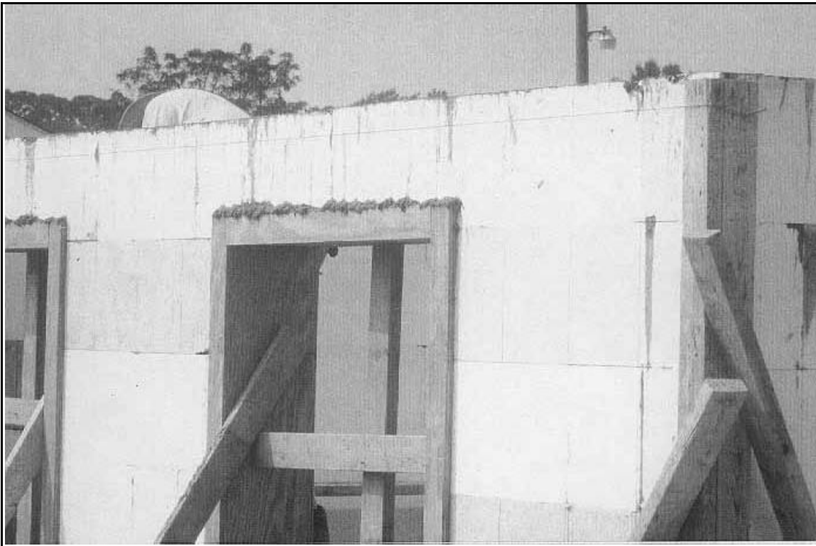
Photo 50: Site #4 - Window and Corner Detail
