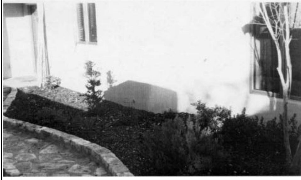
Photo 24: Slab Edge From Outside Under Natural Conditions
