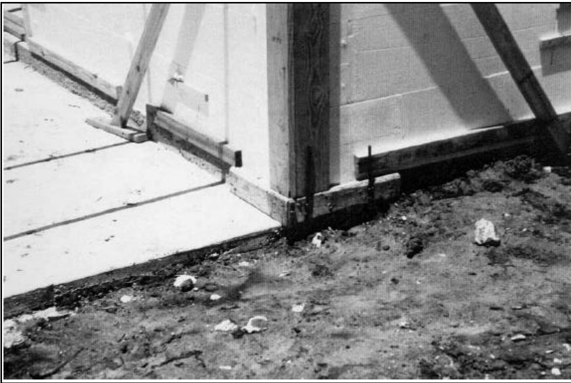
Photo 4: Site #1 - Corner Detail
