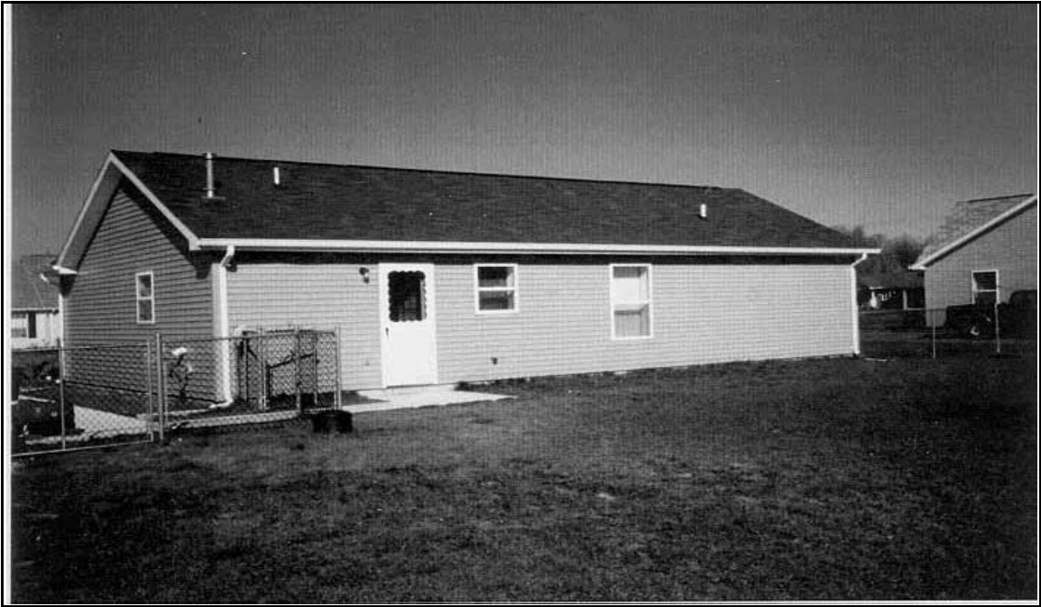
Photo 46: Site 4 - Rear Elevation
