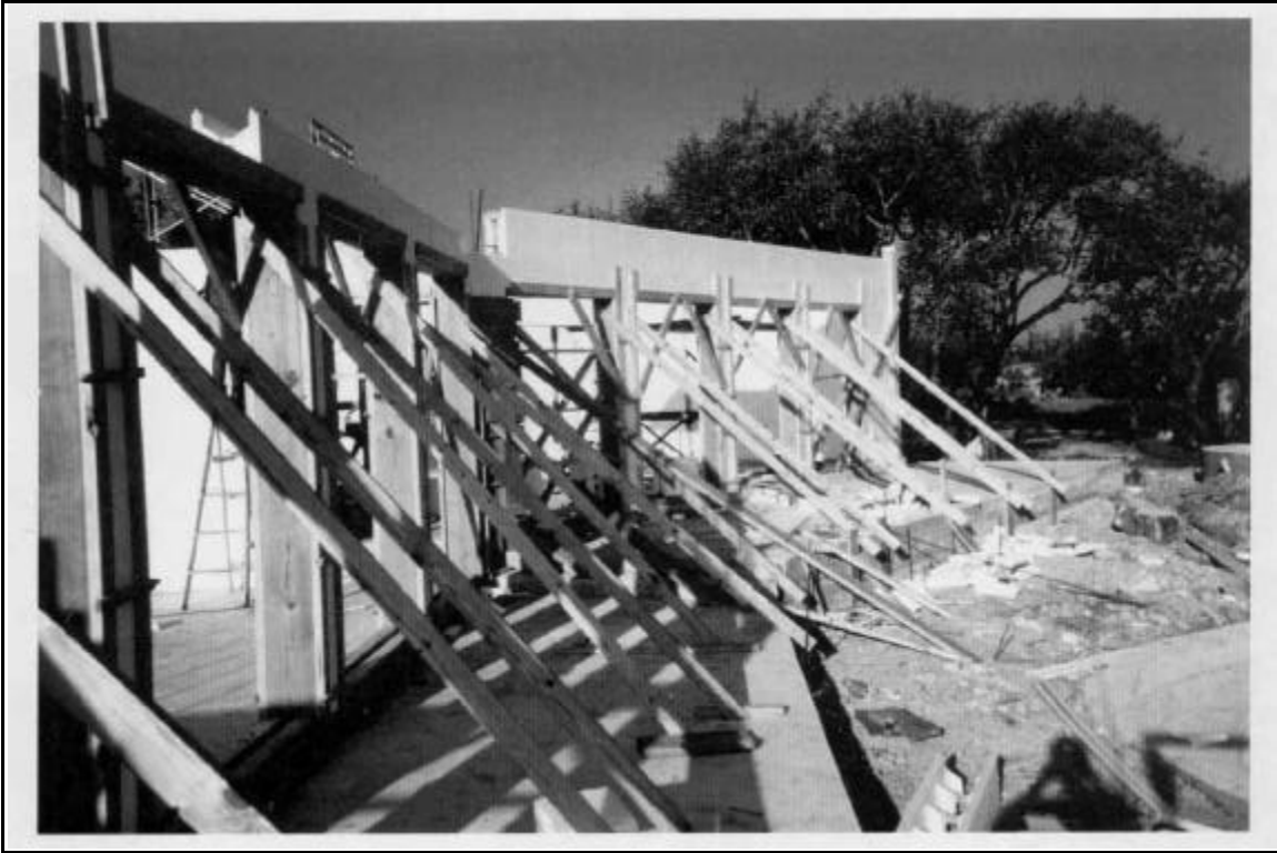
Photo 17: Site #2 - Bracing of Full Length Window and Door Openings
