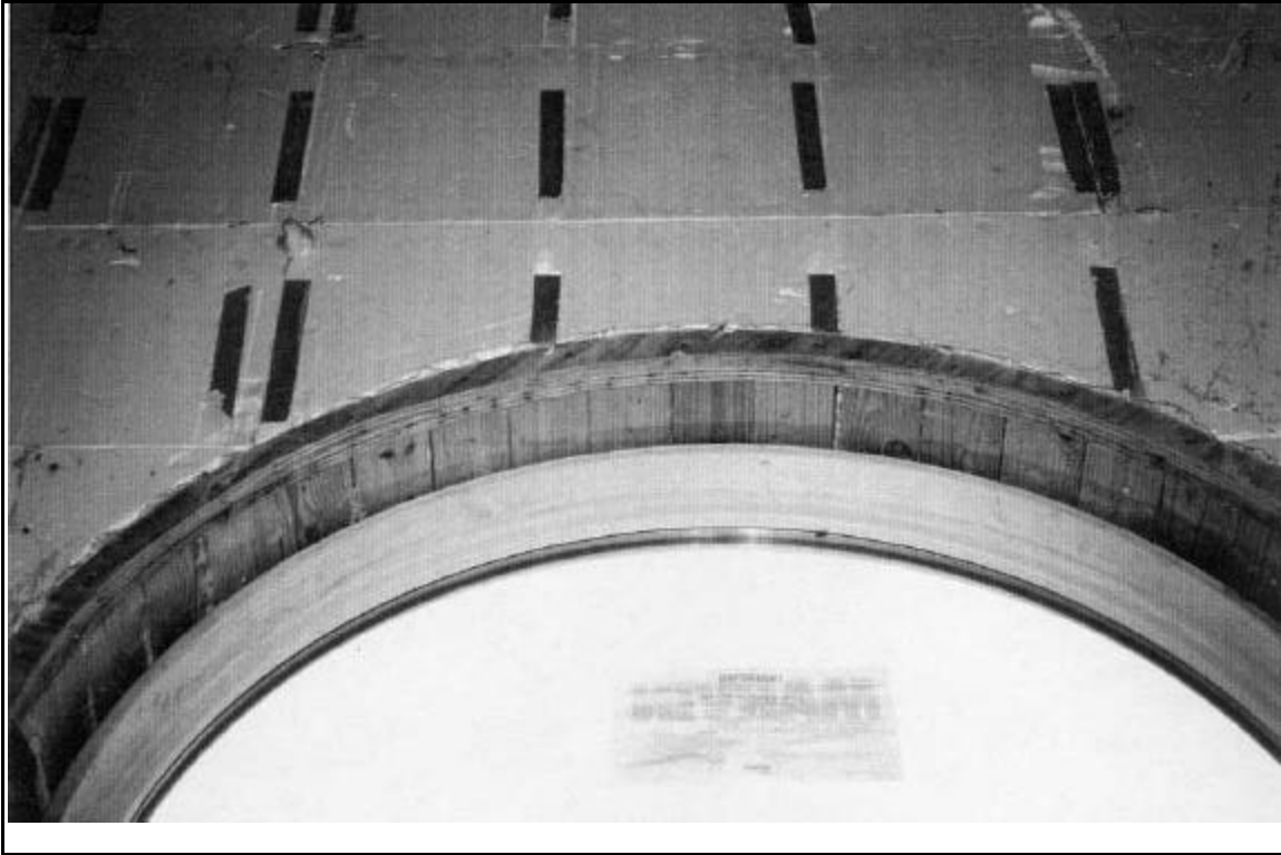
Photo 9: Dominion Building Group Site - Curved Window Detail - Cut Forms
