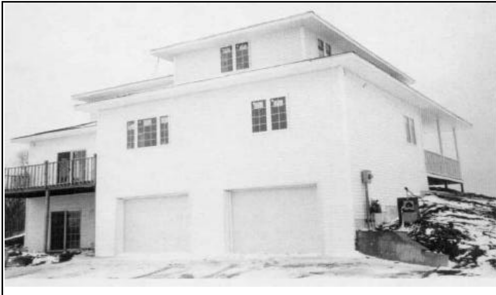
Photo 27: Site #3 - Rear Elevation
