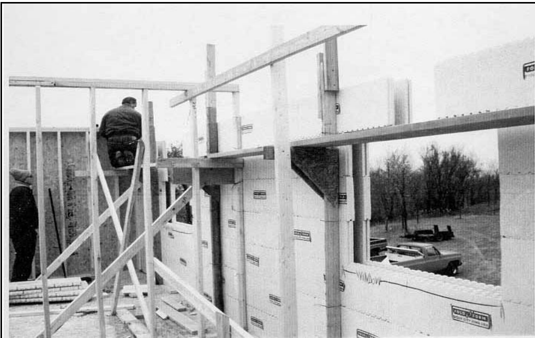
Photo 32: Site #3 - Second Story Wall
