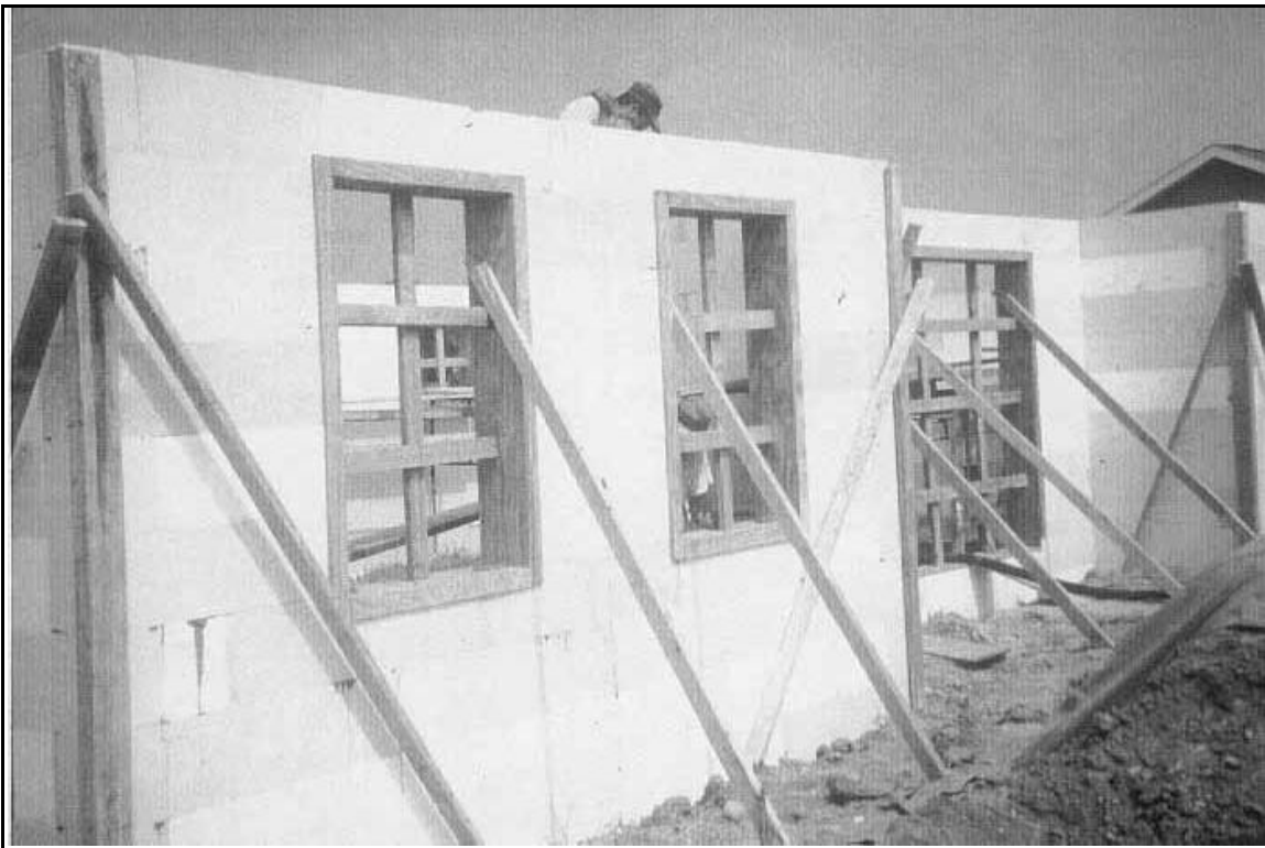
Photo 48: Site #4 - Bracing of Reddi-Form Wall
