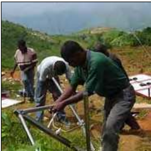
Equipment installation at Radio Eko in Pilate.
