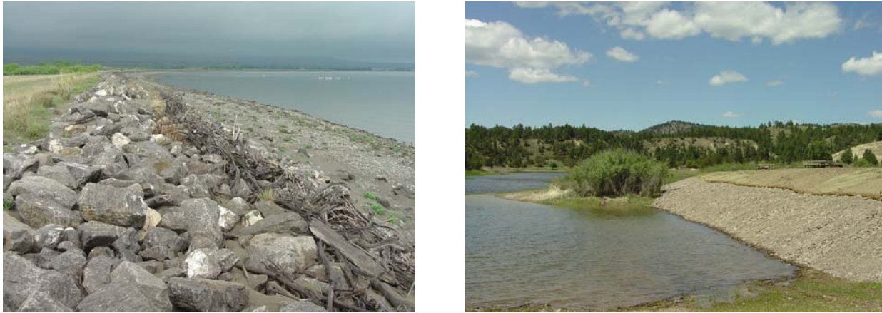
Figure 6. Examples of riprap at Canyon Ferry Reservoir.
