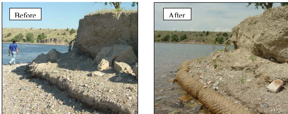
Figure 3. Cave Point is a site where Reclamation has implemented and is monitoring shoreline stabilization measures including a coir log and cottonwood/willow plantings.
