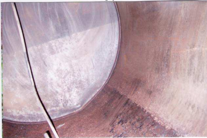
Photograph of the used oil underground storage tank after cleaning.
