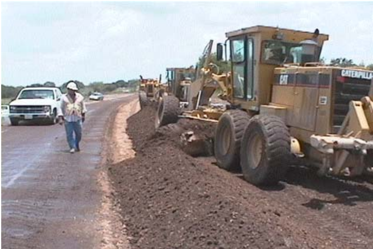
Figure 7-4 Blade Mixing Operation
