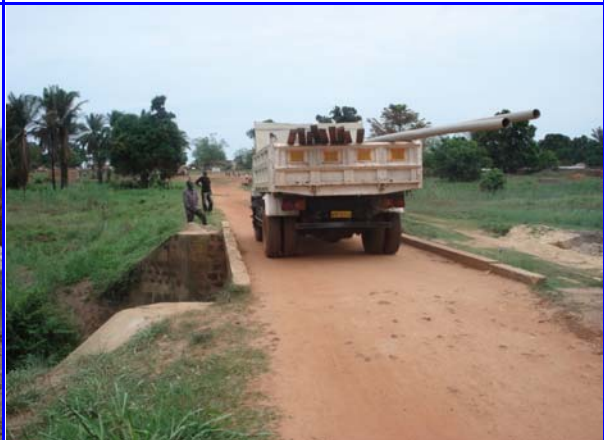
One of the Bridge in Good Condition
