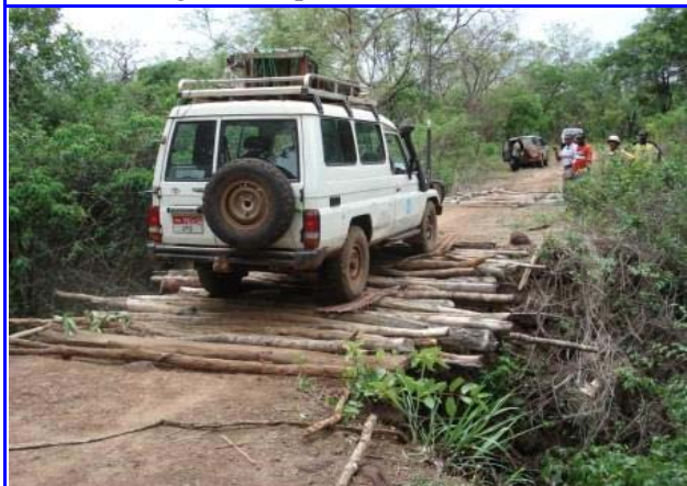
Bridge in Dangerous Condition
