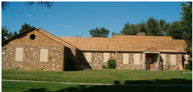
One of the Stewart Buildings Receiving a New Roof
