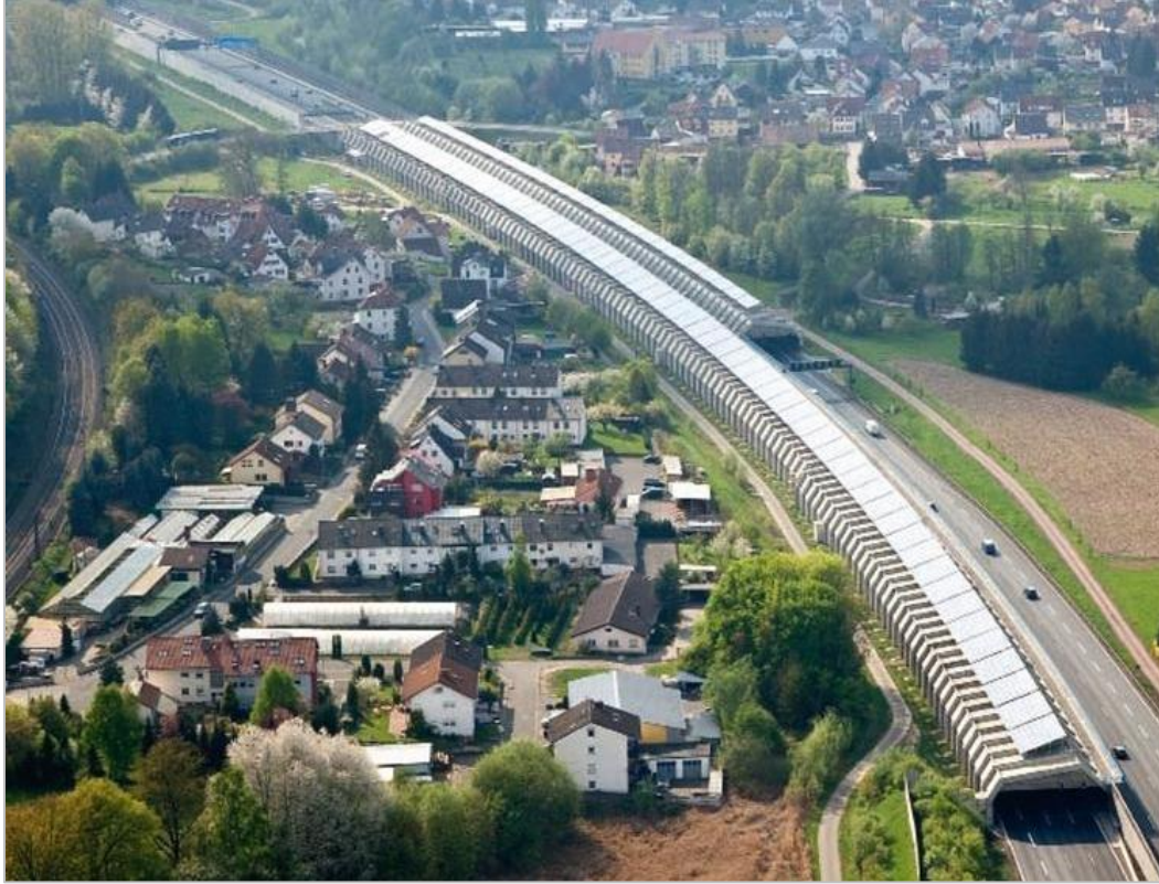
Figure 3: The German Unity Motorway Planning and Construction Company constructed a 2.8-megawatt (MW) solar array on the roof of a 2.7 km long noise-barrier tunnel on the A3 highway near Aschaffenburg, Germany.
