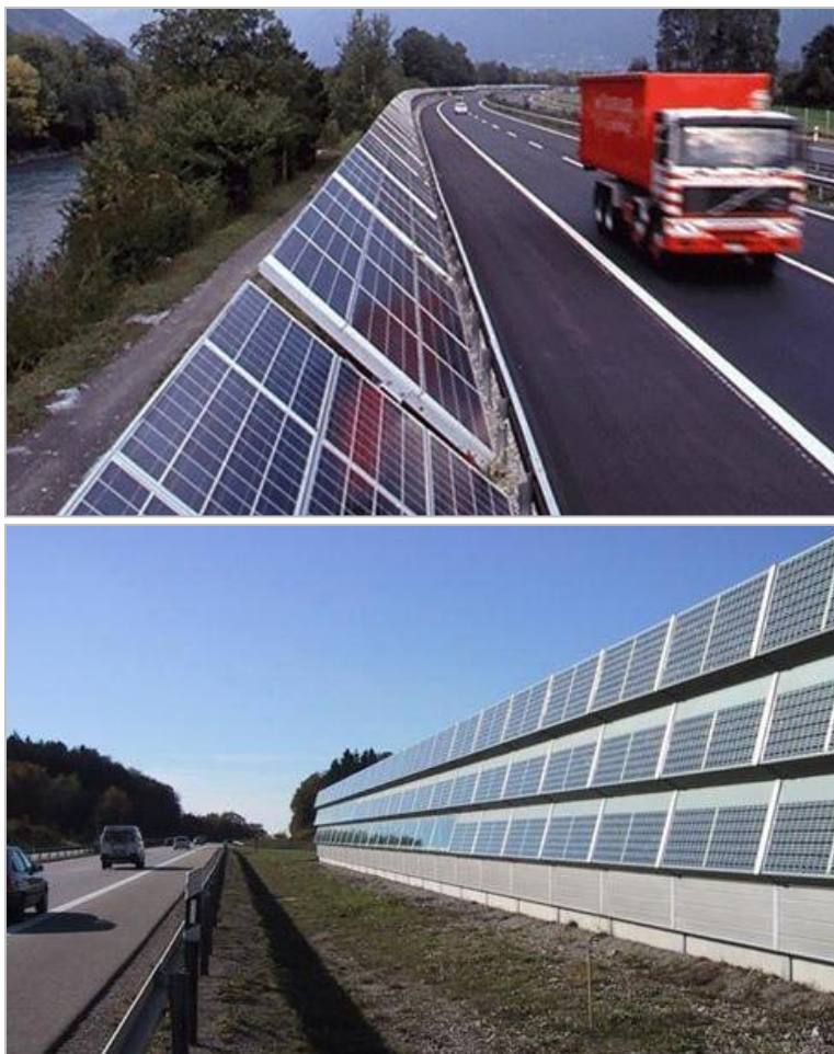
Figure 2: PV sound barrier in Friesing, Germany (top) and PV system mounted on a noise barrier (bottom)
