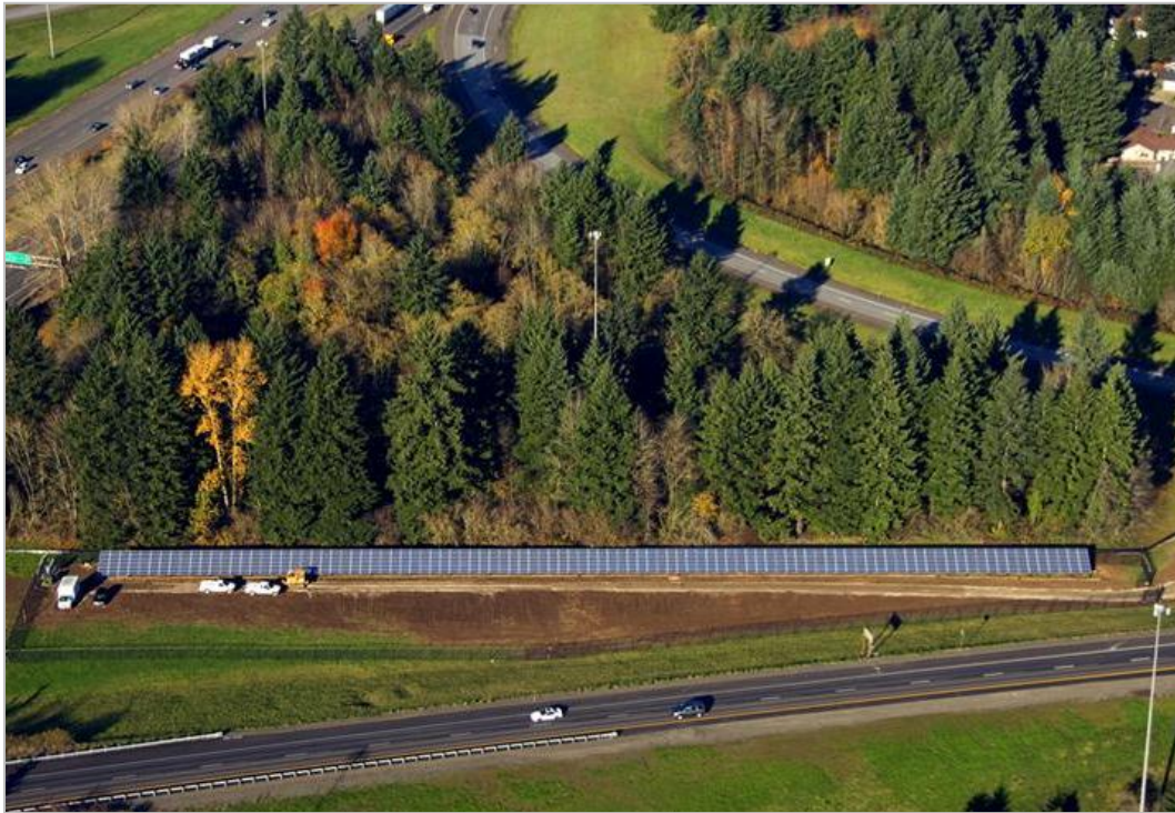
Figure 4: Aerial view of Oregon DOT's Solar Highway Demonstration Project Photo credit: Oregon DOT
