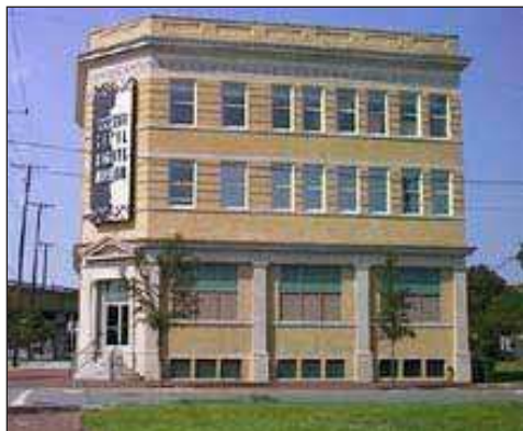
The Ralph Mark Gilbert Civil Rights Museum in Savannah, Ga., will lower its annual electricity costs by an estimated $7,000 thanks to new lighting from PureSpectrum, Inc.
