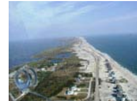
Heading north from the village of Rodanthe, North Carolina, Highway 12 appears as a fragile vein running through Pea Island National Wildlife Refuge. FWS Photo.
