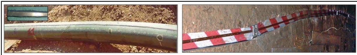
Figure 4: Examples of distributed sensing cables installation (a) full bonding and (b) clamping.
