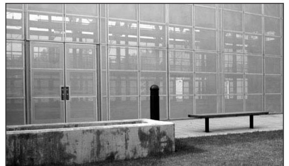
The Williamsburg Community Center, Brooklyn
