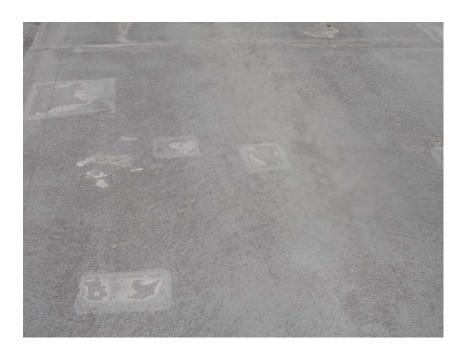
The deteriorated concrete slab at the northeast Garage entrance is shown to the right. The previous patches are beginning to fail.
