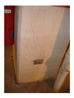
Slab settlement and differential movement occurred in South Garage Level 1 as shown here. This has created a tripping hazard.
