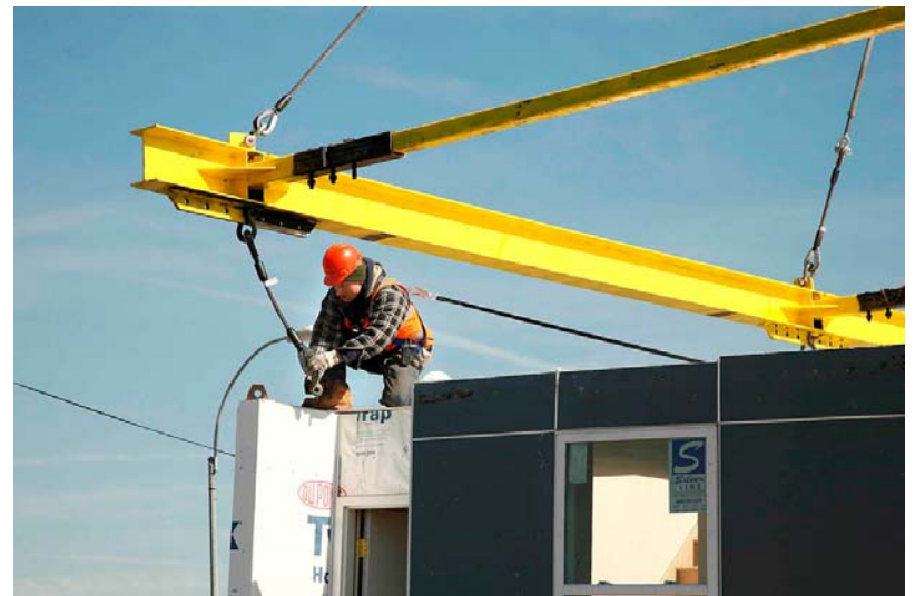
HPD Contractors hard at work
