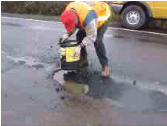
Figure 4.5: Installing TAG 8000 into a pothole with standing water at Century Drive
