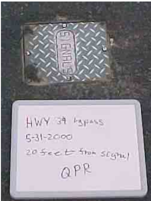
Figure 4.7: Metal signal plate prior to patching
