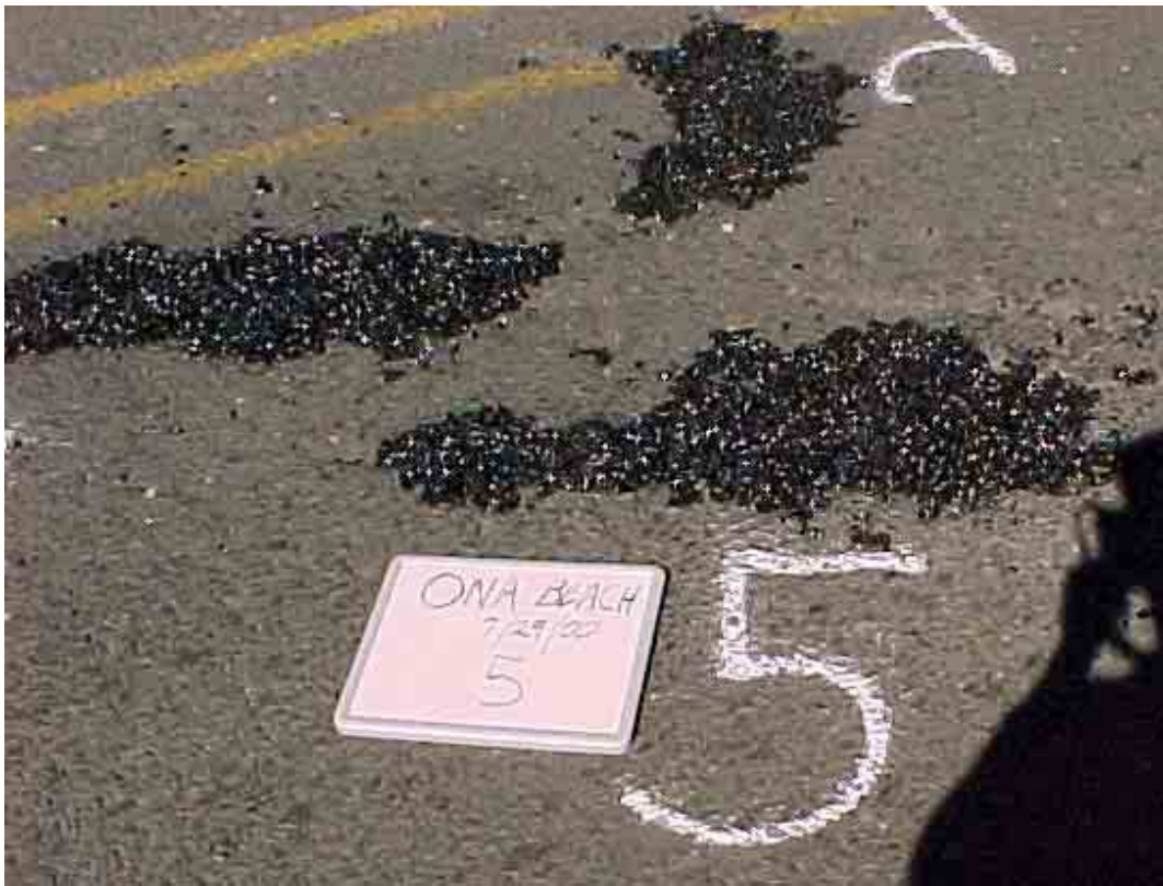
Figure B.2: Three Ona Beach patches prior to compaction
