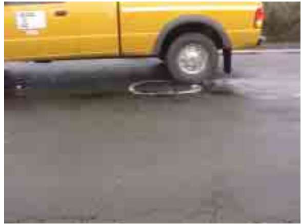
Figure 4.6: Using a truck for compaction
