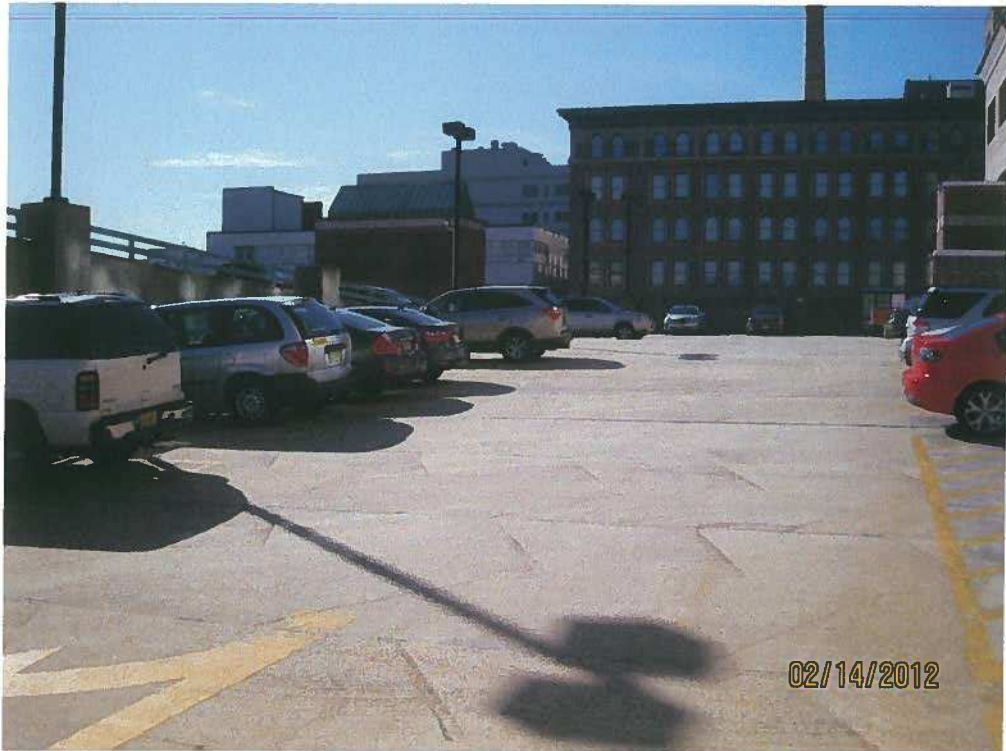
View of 5th Level of Parking Garage EXHIBIT 'C'
