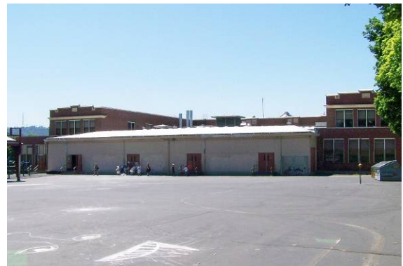
Main building (143A), looking westward.
