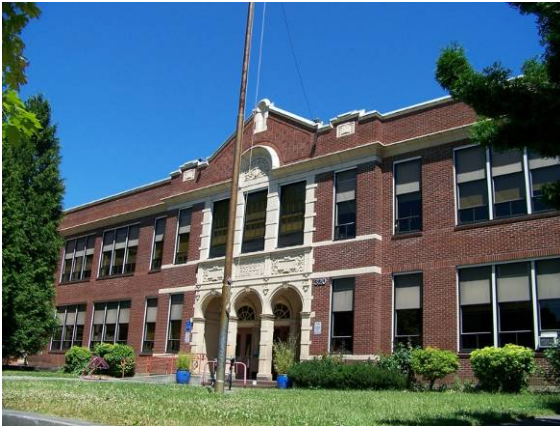
Main building (143A), looking northeast.
