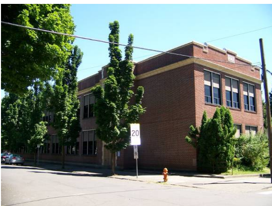
Main building (143A), looking southeast.
