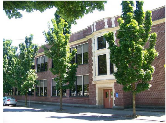
Main building (143A), looking southeast.
