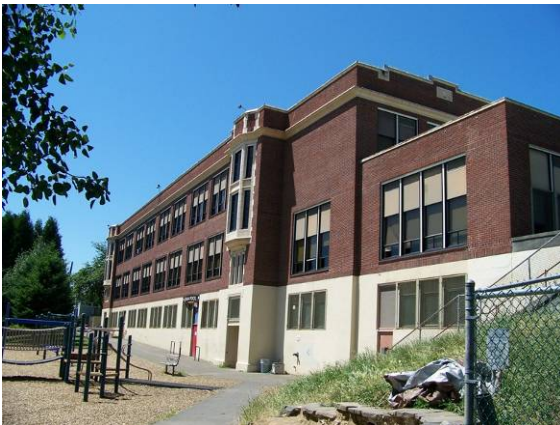
Main building (143A), looking northwest.
