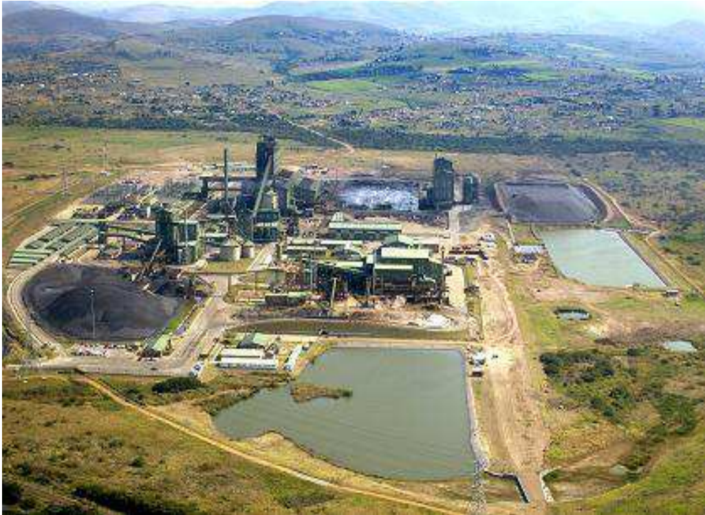
Aerial of Central Processing Plant at Empangeni
