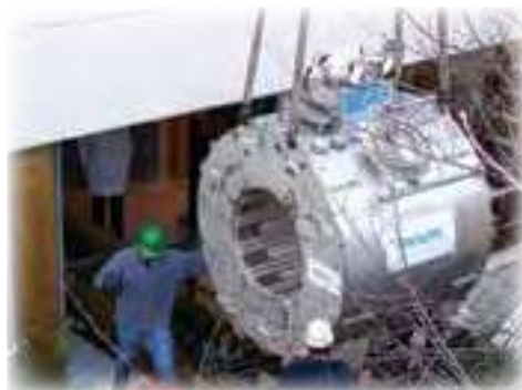
A crane and specially built ramp were used to lower the 1.5T Philips Magnet into place.
