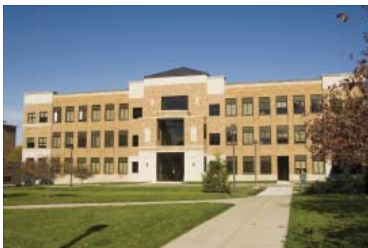
Stalker Hall renovation on quad side
