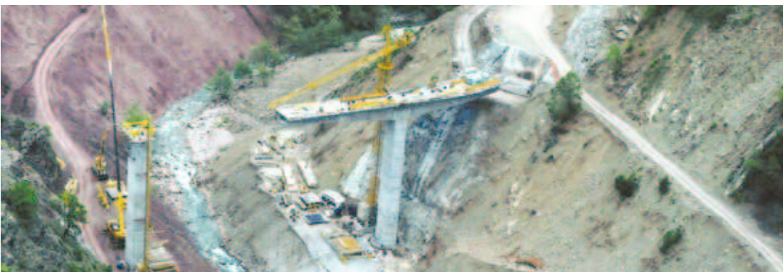
Energy Production works, Mesochora Road Tunnel, Bridge of Nea Pefki
