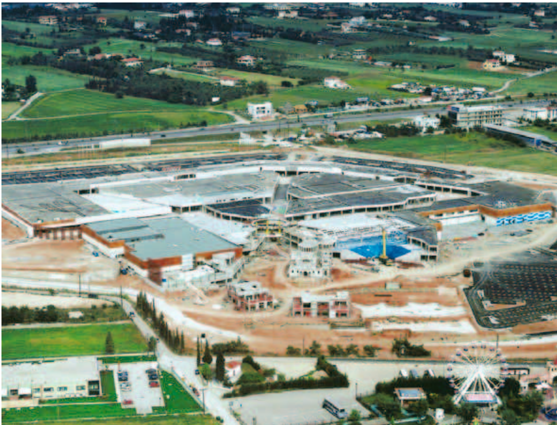
Construction of shopping and entertainment centre "Mediterranean Cosmos" in Pylaia, Thessaloniki
