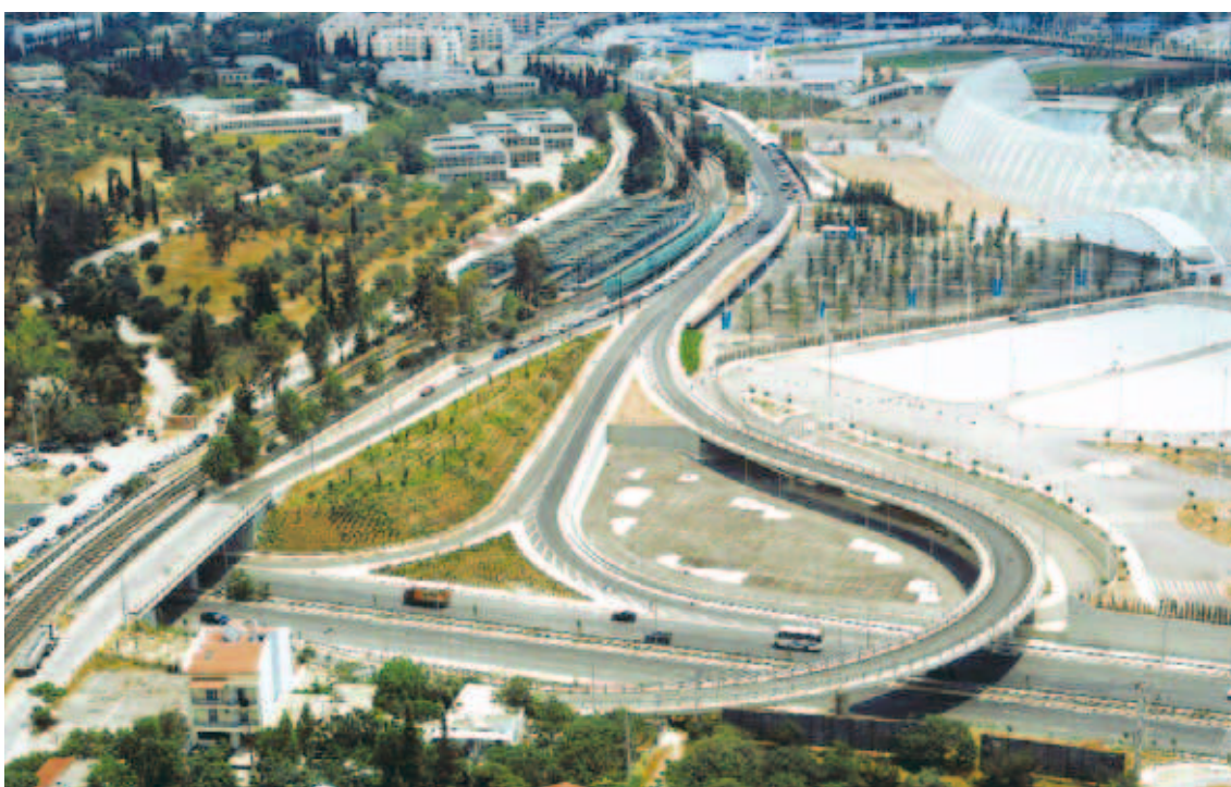
Roadworks around the Athens Olympic Sports Center
