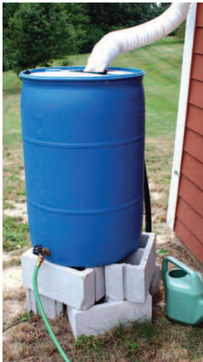
From the sky to roof to tomatoes * This barrel captures and stores rainwater for use in MTSO’s Community Garden
