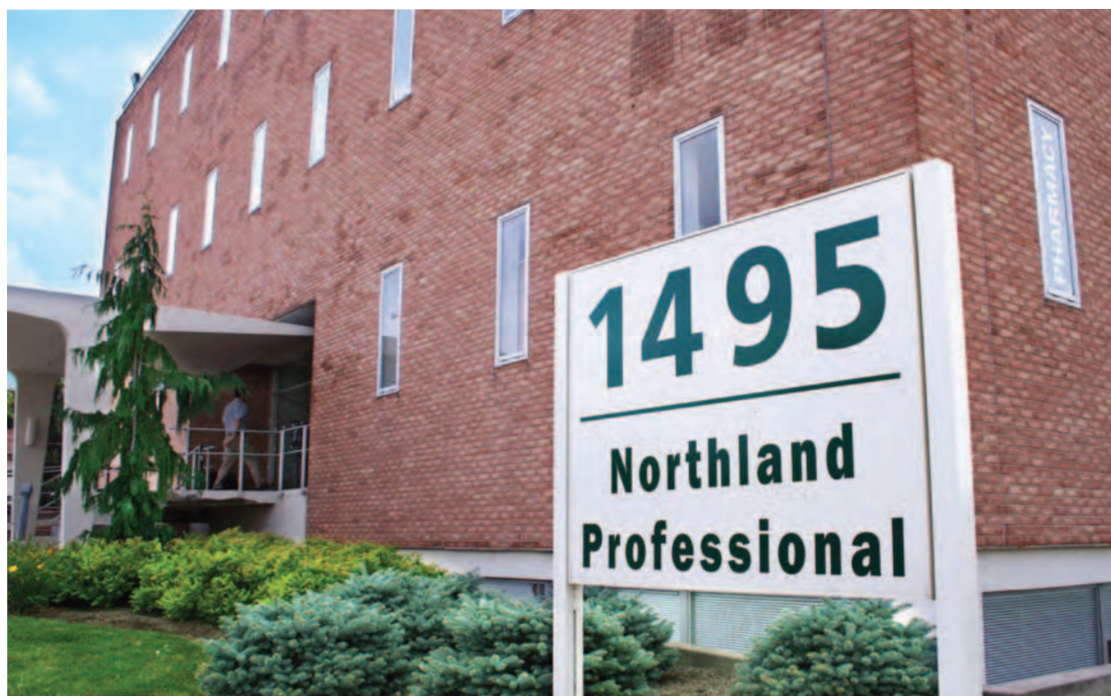
A firm foundation ✱ The Morse Road professional building given to MTSO by the Masons in June
