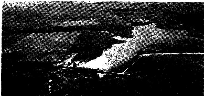
Yanktonai Dam and Reservoir
