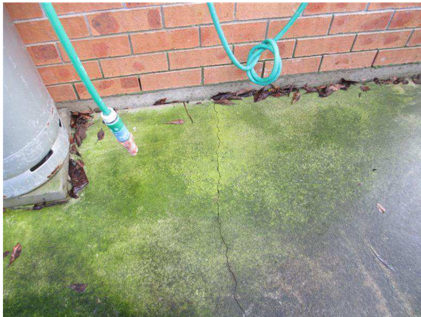
Figure 4 - Minor crack in pavement on southeast side
