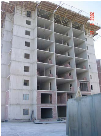
Figure 10: A Typical Tunnel Form Building Nearing Completion (Note Masonry Facade Elements)
