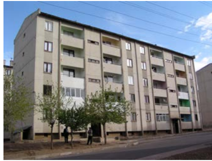
Figure 20: A Practically Unscathed Building Subjected to the Bingol Earthquake
