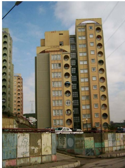
Figure 17: The Post-Earthquake Condition of Another Tunnel Form Building of a Different Housing Complex in İzmit
