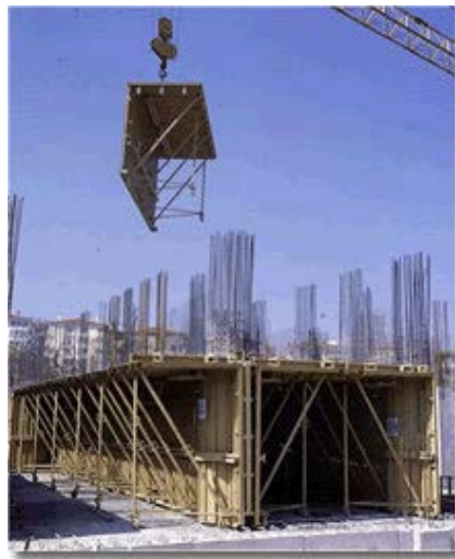
Figure 8: An Application of Half-Tunnel Forms
