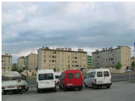
Figure 19: Tunnel Form Buildings after the Bingöl Earthquake of May 1, 2003
