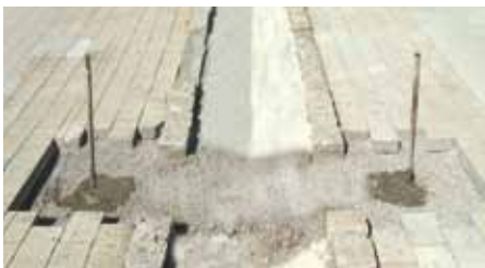
Completely installed injection piles
