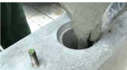
Grouting of the foundations
