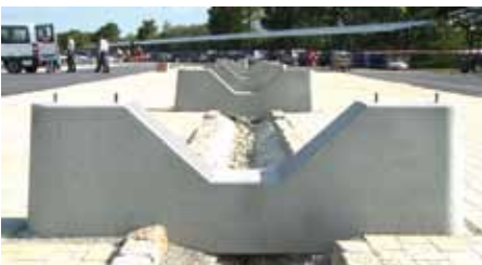
Readily installed and levelled pre-cast foundations
