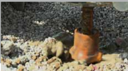
Injection of cement mortar using the drill bit
