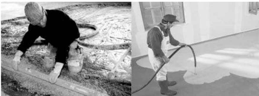
Fig. 7 Placing of “non-slump” cement-based floor screed (left) and flowing anhydrite-based floor screed (right).
