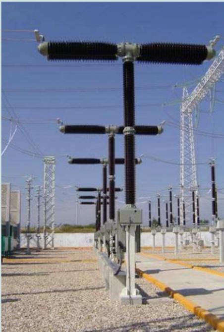
3AP2 FI 420 kV Live-tank circuit-breaker in operation at a major power transmission and distribution company
