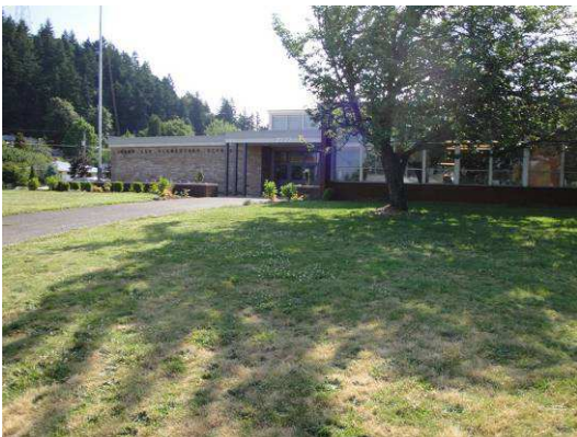
West elevation front entry
