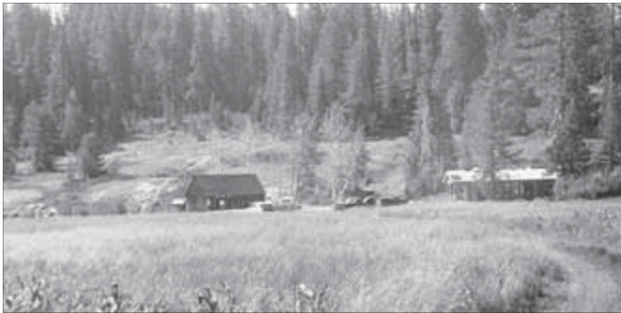
For a short time the swimming pool was flanked by two bath houses, east and west of the pool. This photograph shows the new bath house (on the right) under construction. Photo, 1962. (LAVO Collection, newbath)
