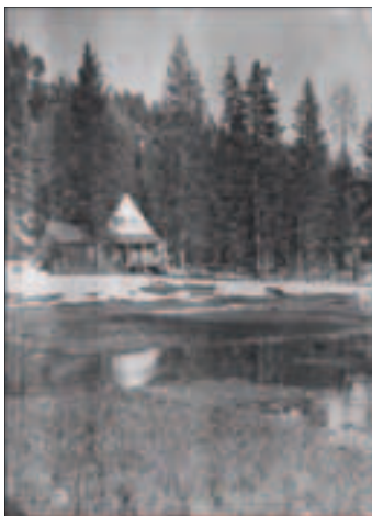
View from the south to the “big house” constructed by Edward Drake across standing water in the meadow. The natural topographic bench provided a dry building site. Fences are visible on the right hand side (east) of the house and Flatiron Ridge is in the background. Photo, circa 1902. (LAVO Collection, 1902cabin)
