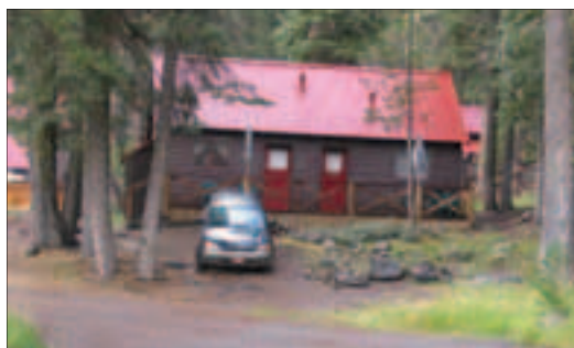
Contemporary view looking west to the Manager's Cabin. Photo, 2003. (National Park Service)
