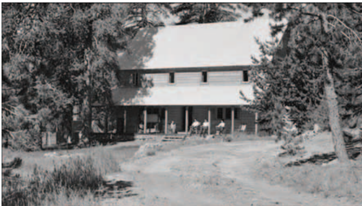
The early path of the Warner Valley Road routed it just east of the lodge. Photo, 1939. (LAVO Collection, B-1028-1)
