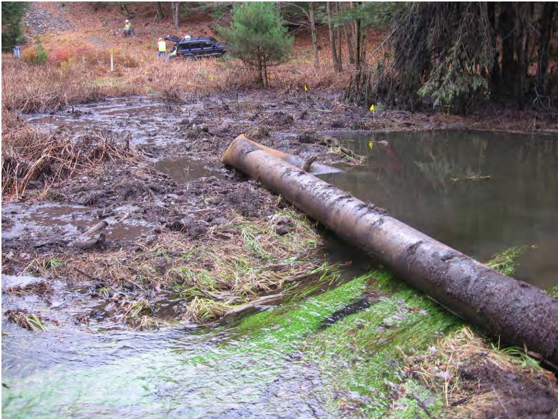
Figure 6: End of 21.7 foot section of pipe in swamp
