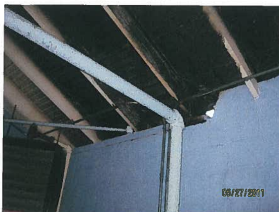
Fire damage to Chapel roof
