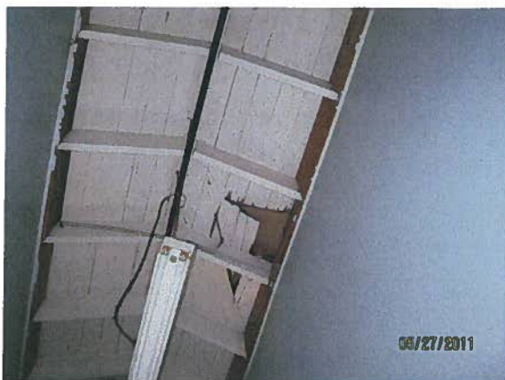
Fire dept. hole punched in Chapel roof
