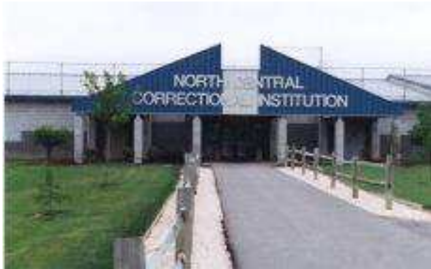
North Central Correctional Institution
