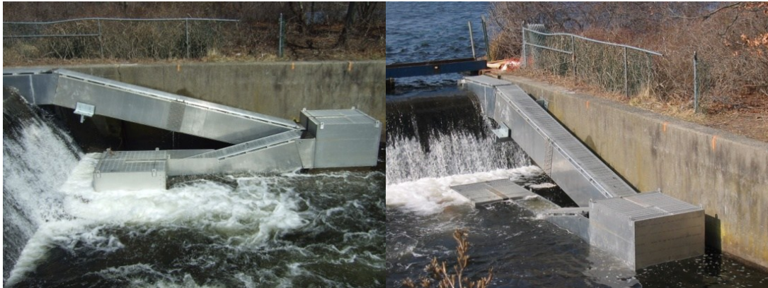
Long Island's first permanent fish ladder, installed March 2008. Hards Lake Dam spillway on Carmans River in Suffolk County's Southern Park, Brookhaven NY This ladder opens up several miles of spawning habitat for anadromous fish, such as alewives and trout. Photo credit: Long Island South Shore Estuary Reserve Office
