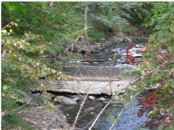
A dam will fail if not maintained. Pictured are 3 views of the first manmade barrier upstream from the Hudson River on the Quassaick Creek (Orange County, NY). The dam before 2006 (far top right) was known to have contaminated sediment in the impoundment. Above are 2 views of the dam after it breached during the 2007 floods. Photo credit: DEC Hudson River Estuary Program
