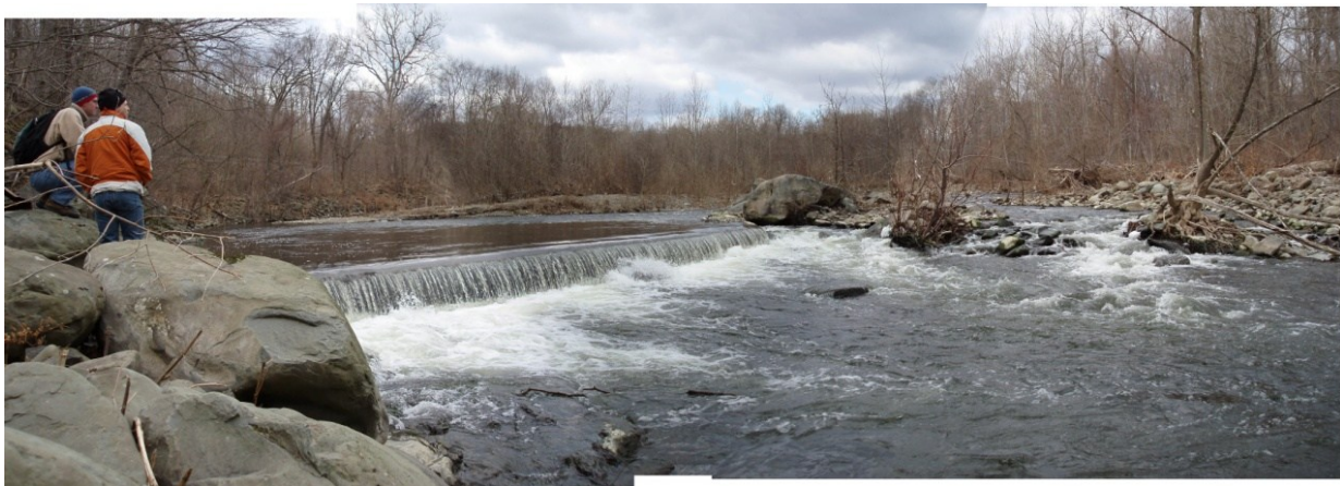
Moodna Creek Dam in New Windsor. Partial first barrier is upstream of Hudson River due to partial breach (right side of picture) from lack of maintenance. The dam has been under consideration for removal (Orange County, NY). Photo credit: DEC Region 3 Hudson River Estuary Program.
