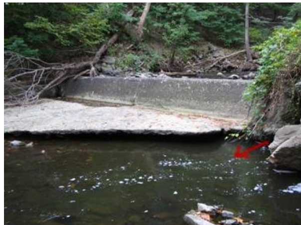
A dam will fail if not maintained. Pictured are 3 views of the first manmade barrier upstream from the Hudson River on the Quassaick Creek (Orange County, NY). The dam before 2006 (far top right) was known to have contaminated sediment in the impoundment. Above are 2 views of the dam after it breached during the 2007 floods. Photo credit: DEC Hudson River Estuary Program
