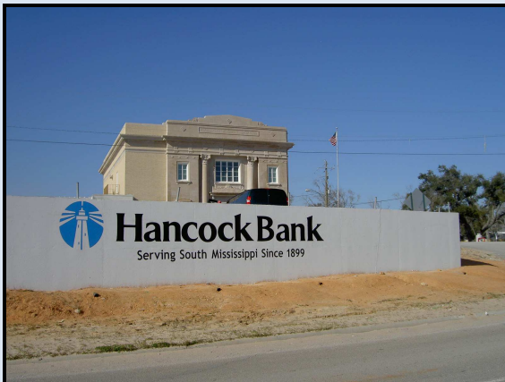
Hancock Bank repair in Mississippi following Hurricane Katrina was based in part on regional commitment and customers in southern Mississippi.
