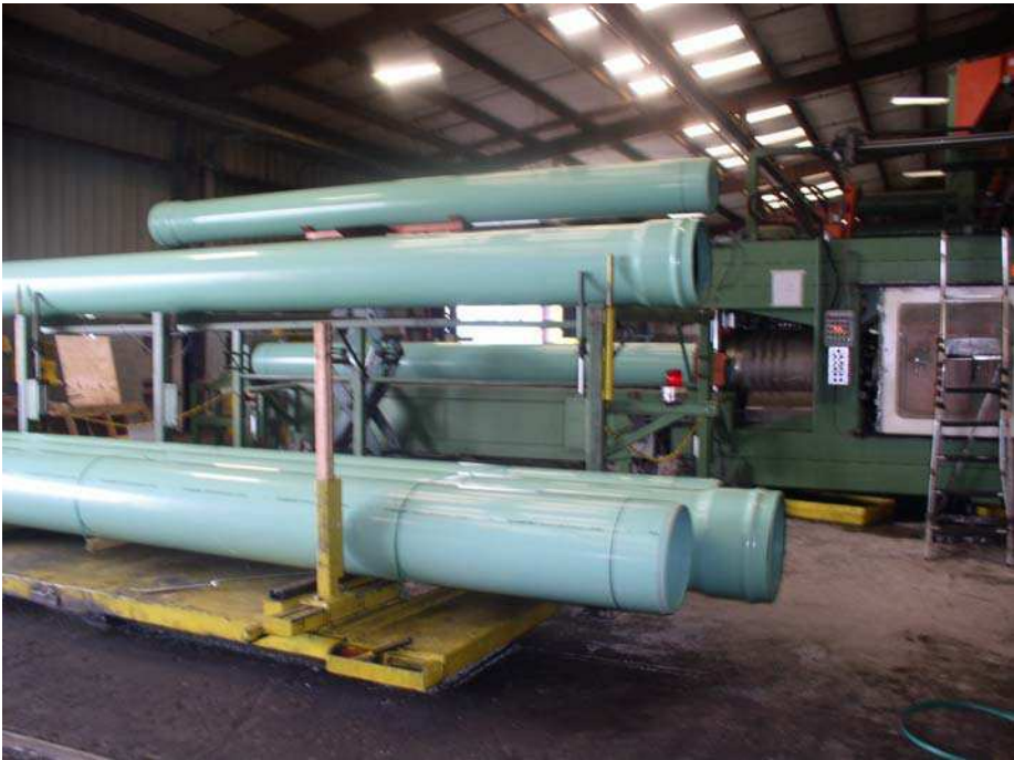
Exhibit 2. The pipe storage rack and unitizing table from a different angle.
