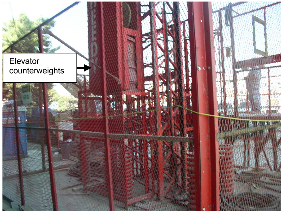
Exhibit 3. A picture of the counterweights at the bottom of the elevator mechanism when the elevator is ascended to the top floor.
