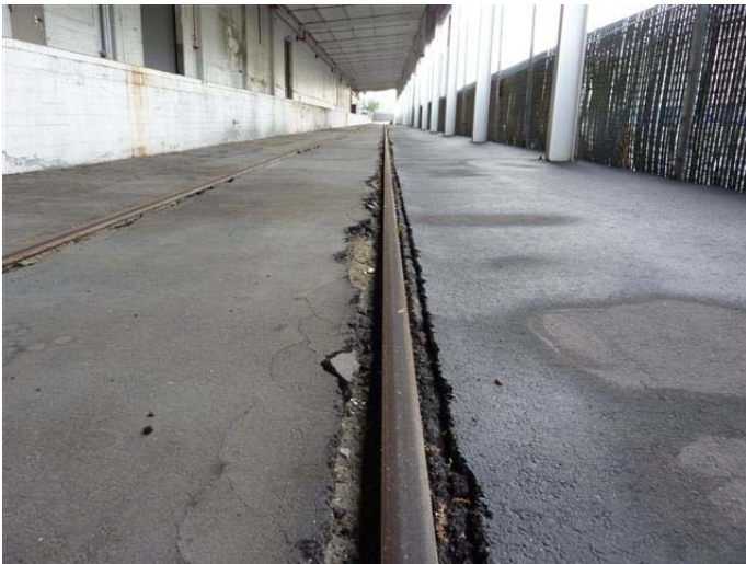
Photo 1. Rail siding very clean
