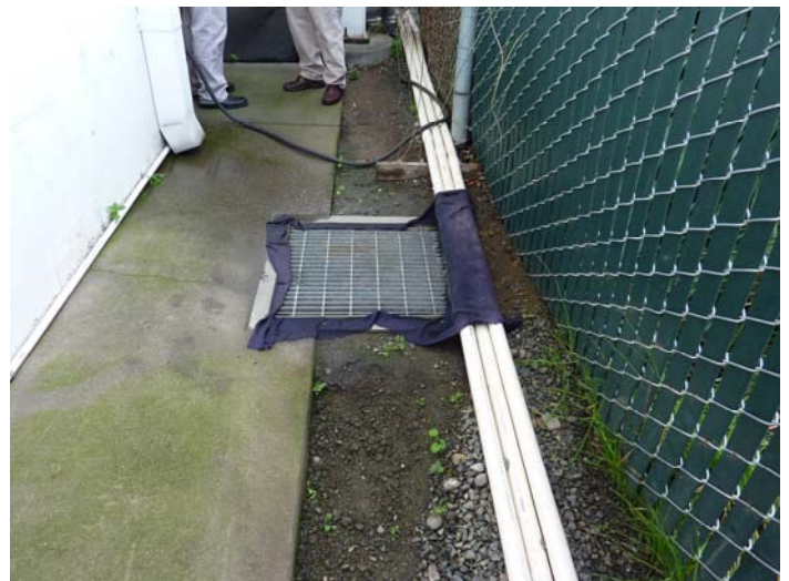
Photo 4. Screened storm drain. Screen very clean
