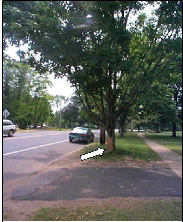
Photo 1 Photograph Showing Site of Impact
