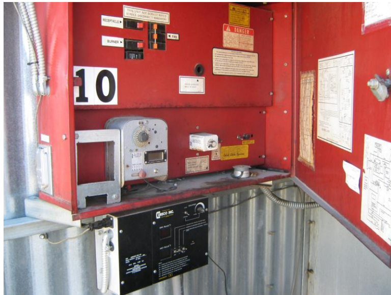
Figure 1-3: Automated curing controller mounted in a tobacco barn
