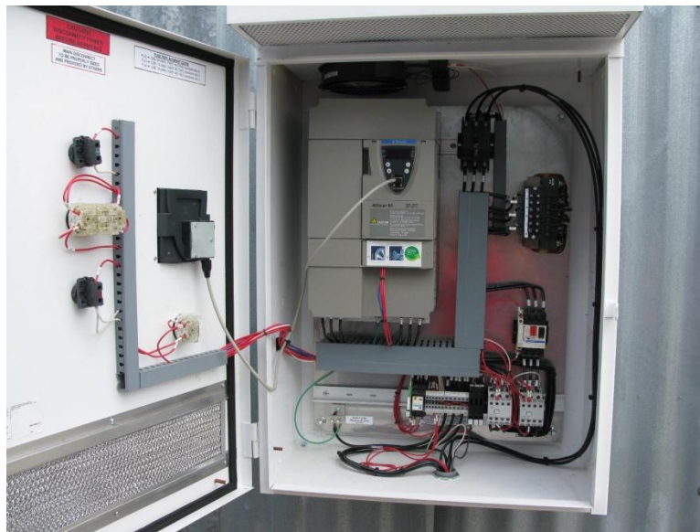
Figure 3-2: Inside of VFD control box, showing the VFD and Line Reactor
