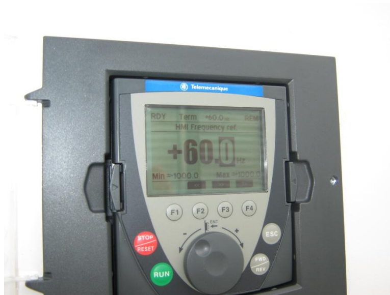
Figure 3-3: Close up of operator interface and frequency display on the VFD
