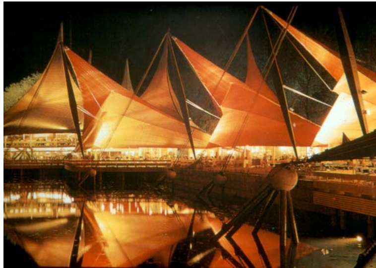
Fig. 3. Anticlastic membrane structures for Expo'64 Lausanne, Switzerland Architect: M.J. Saugey and G.G. Schierle; Frei Otto, consultant
