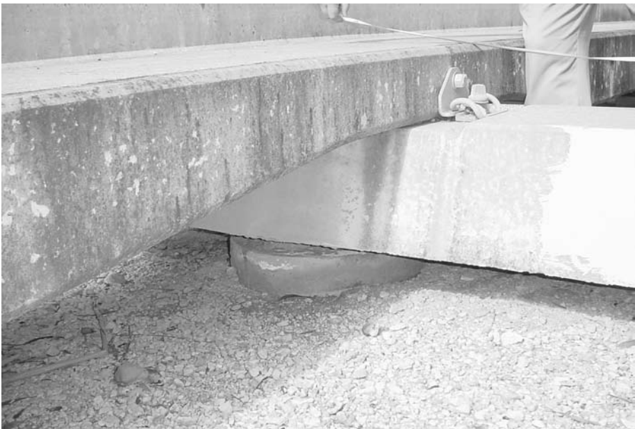
Figure 9. Precast concrete construction
