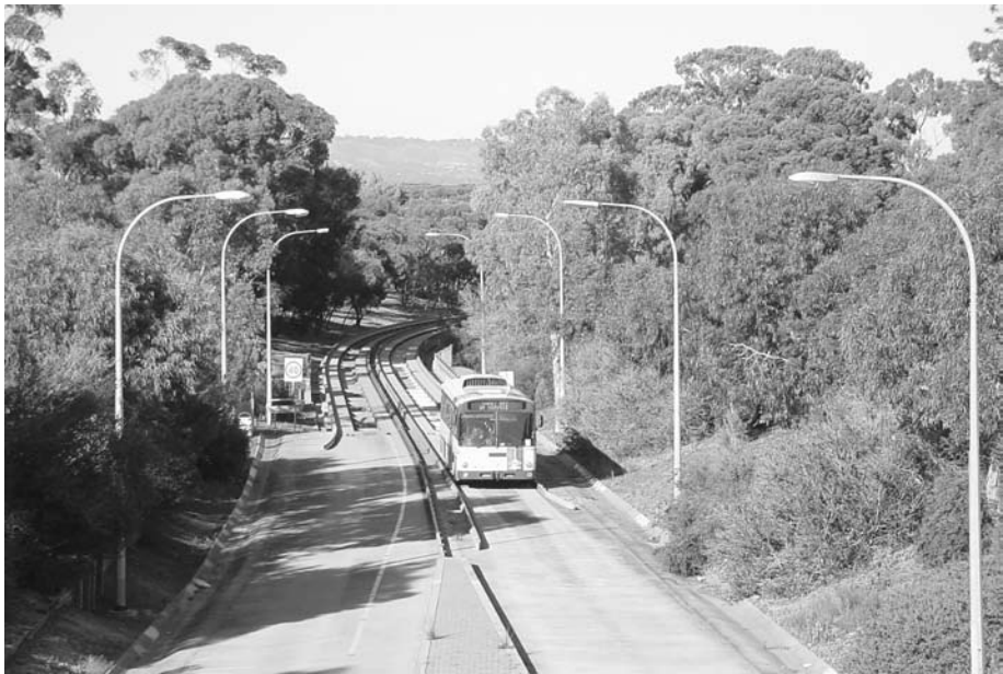
Figure 4. CGB guideway entry funnel, Adelaide
