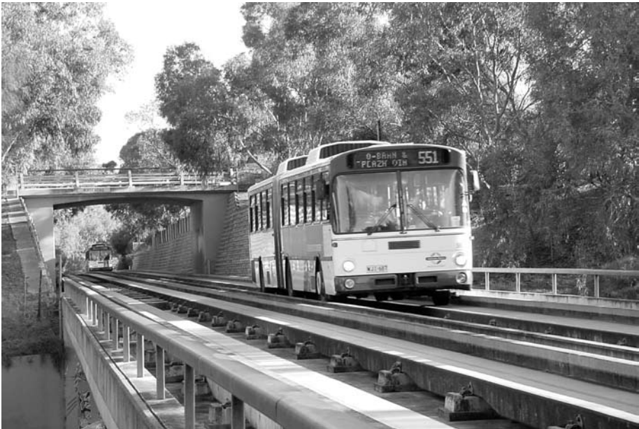
Figure 1. Curb Guided Bus, Adelaide
