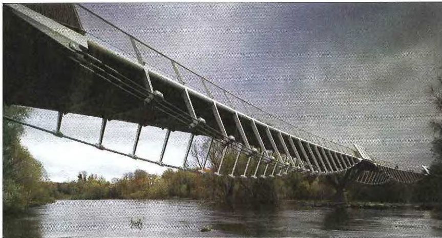
The Living Bridge crosses the River Shannon and connects two parts of the Limerick University campus. Its six identical spans are supported by below-deck edge-cable trusses (above). Each segment of the C-shaped crossing widens at pier locations, creating a pulsing rhythm over the river (left).
