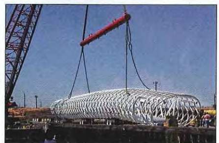
The main span of the pedestrian bridge at Seattle's Museum of Flight is made of pipe bent into pure circles but has an elliptical section (top). Fabricators completed assembly in Tacoma (right) and transported it to the site in one piece.
