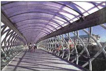
The main span of the pedestrian bridge at Seattle's Museum of Flight is made of pipe bent into pure circles but has an elliptical section (top). Fabricators completed assembly in Tacoma (right) and transported it to the site in one piece.
