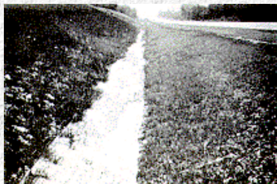
Figure 10. Installed Jute Net Channel Lining
