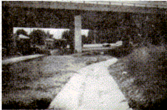
Figure 1. Rigid Concrete Channel Lining
