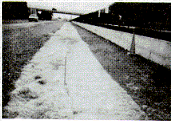
Figure 14. Installed Curled Wood Mat Channel Lining
