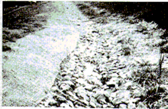
Figure 2. Composite Channel Lining (riprap and jute net)
