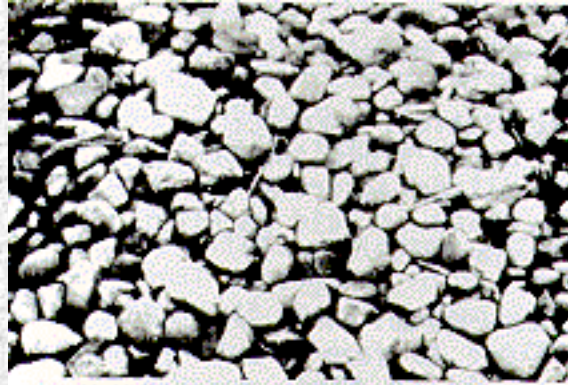
Figure 6. Gravel Channel Lining
