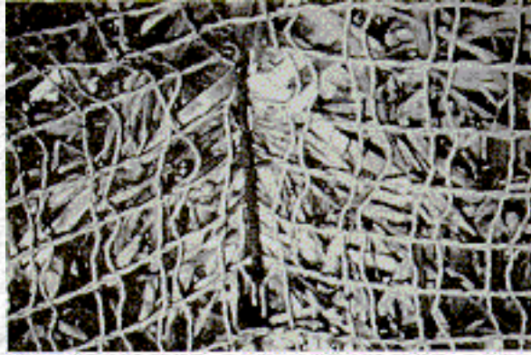
Figure 17. Straw With Net Channel Lining
