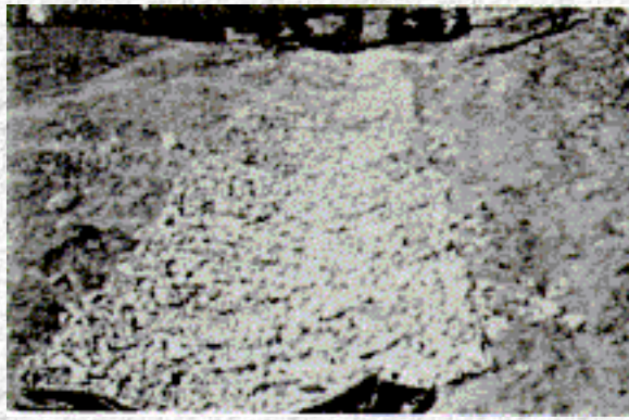
Figure 5. Wire-Enclosed Riprap
